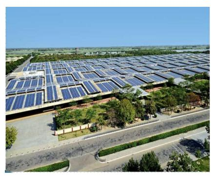
L&T in Punjab having Largest Roof Top Plant in the World - 7.52MW with more than 30,000 PV panels and Power from the plant being fed to the local grid through a PPA signed with the state distribution company
